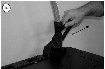
Step 4: Reattach the hook and loop at the top edge of the fabric sleeve. Pull the hook and loop cinch tie tight around the cable bundle. Wrap cinch tie around the cable bundle and attach it to itself. If applicable, trim off the excess cinch tie material.
