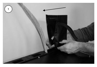
Step 1: Disengage the hook and loop cinch tie and the hook and loop strips along the top edge and side of the fabric sleeve. Open the fitting to accept the existing cable bundle by separating the end of the fitting assembly.
