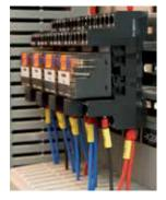
Robustness is also a key parameter for CLT devices, including the CLT01-38S4, which operates with all types of sensors compliant with IEC 61131-2, type 1 and 3, with a 2.35 mA limited current, and type 2, using two inputs per sensor with the correct  $R_{\text{pcc}}$ .
